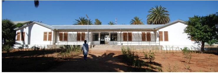
The new ENT-out-patient-department in the Orotta-Hospital in Asmara
